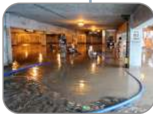
Dewatering of Basement Water
